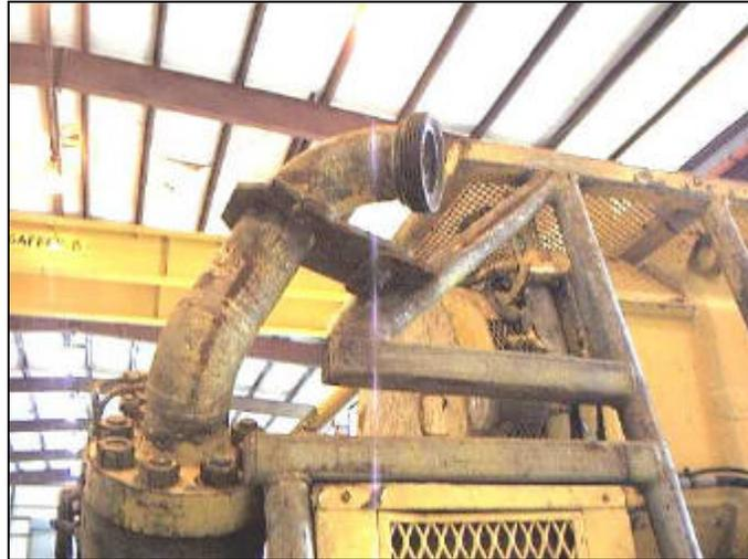
**Figure 7-Insufficient Support**
